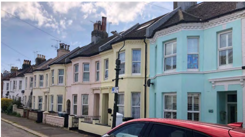
Figure 6: Photo of inappropriate PVCu casement windows
