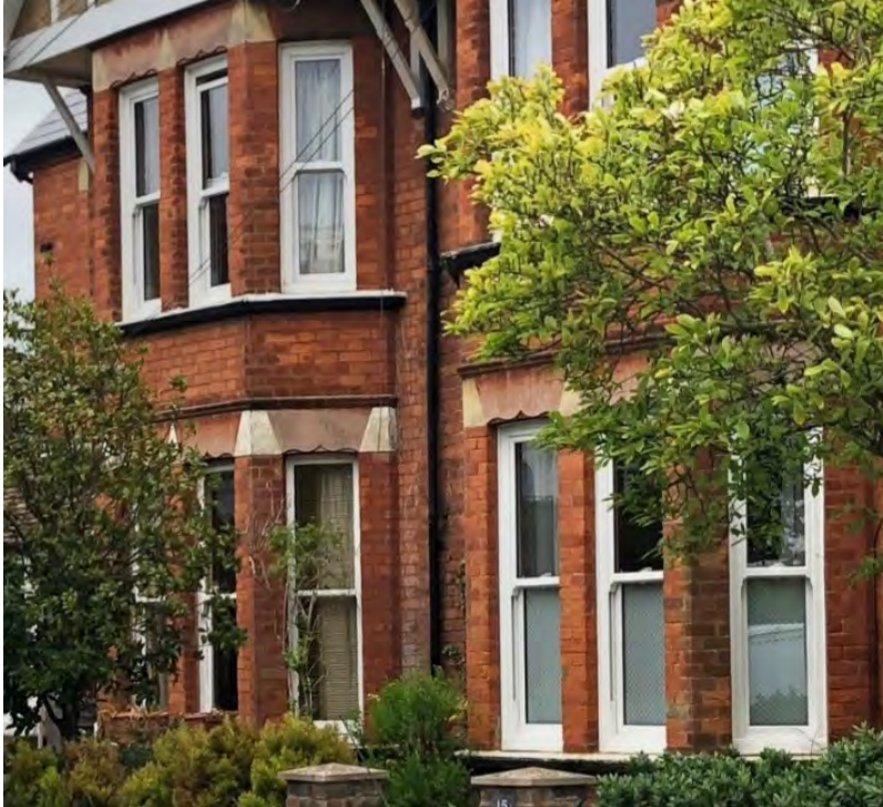
Figure 5: Photo example of timber and PVCu variation in proportionality
